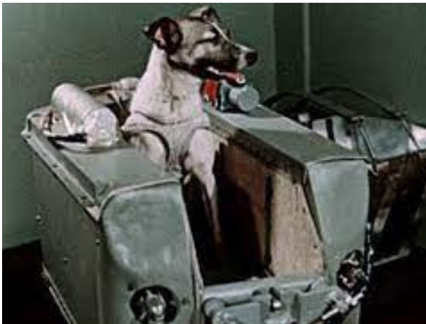
The first inhabited space capsule is launched by the U.S.S.R. Sputnik II carried a dog named Laika, who perished on the fourth orbit from overheating caused by an air conditioning malfunction.
